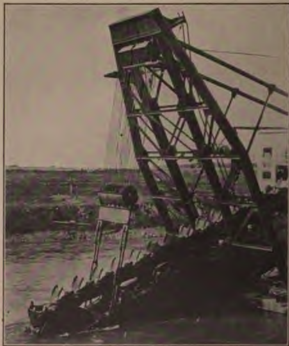
Bucket Chain and Gantry of Ladder Dredge.
